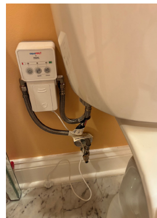
Toilet leak detectors are being installed to save water and reduce flooding.
